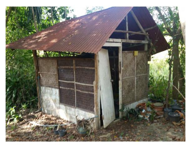
**Building #1**Condition – Collapsed roof / Structurally Unsound / Full of Trash / 3 Broken Toilets outside
